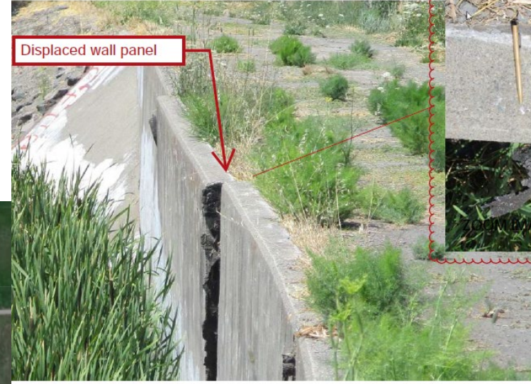
PHOTO 2: Wall 1 Failed Concrete Panel
